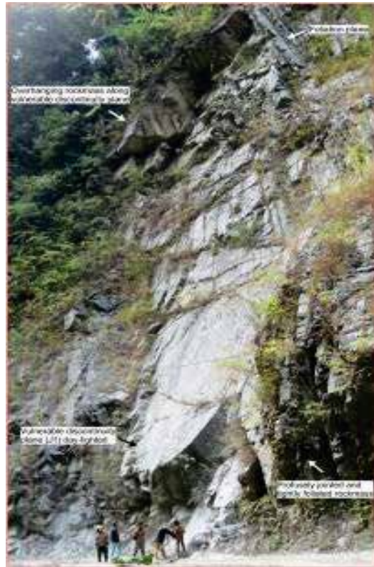
Figure 2 Prominent vulnerable discontinuity
