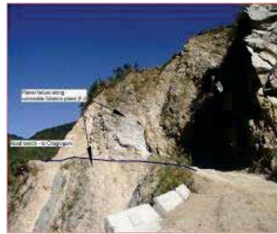
Figure 6 Perspective view of rockslide, visible prominent vulnerable discontinuity plane
